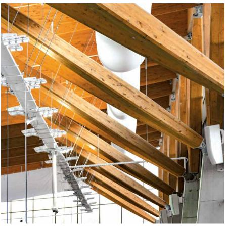
"With the execution of the Stromlo Leisure Centre we have implemented the longest spanning glulam roofing structure throughout Australia. From the very beginning this project had a role model effect. Static properties, design, durability, and sustainability of the natural material wood convince more and more clients in Australia. It seems that we not only have put our finger on the pulse of time but that we are also setting trends."
