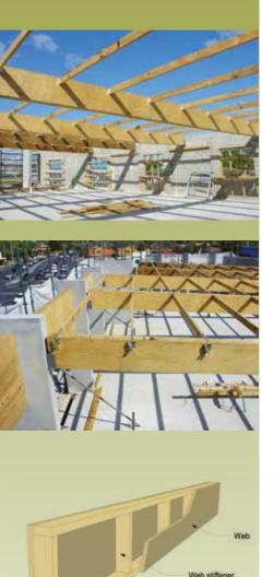
Flexible and lightweight, plywood box beams are a high-strength timber product that can be used in a vast range of residential, industrial and commercial design and building projects.
