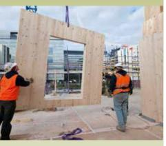
CLT wall panel installation at the Forte project in Melbourne
