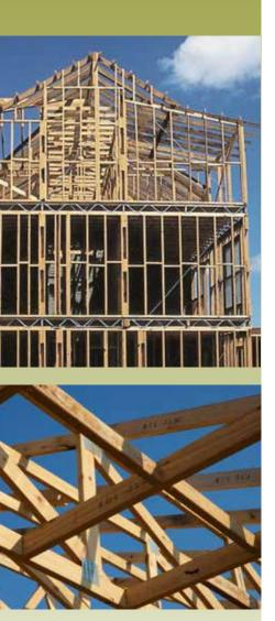
Structural Softwood is the most cost-effective, environmentally beneficial building material for house framing. Its ease of cutting and connection, as well as compatibility with other common housing materials, makes it ideal for this use.
