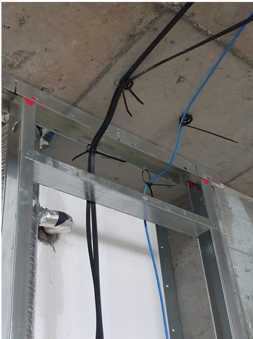
The Vortex Segmented Rebate Track fixed to the concrete.
