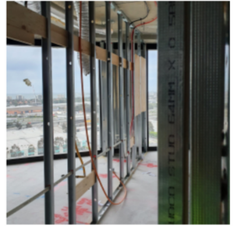
Studco Stud and Track Framing forming an internal wall.
