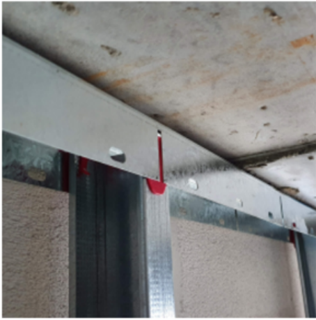
A closer look at the Vortex Isolation Clips disallowing steel-on-steel contact.
