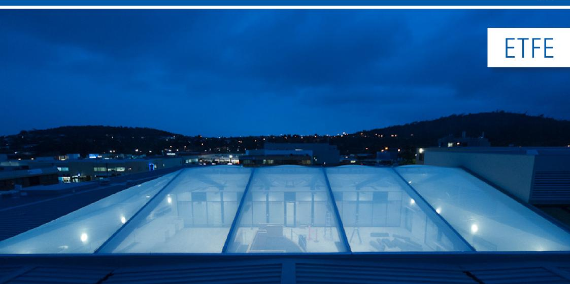
A new generation material, providing an architecturally innovative option, which goes beyond glass Is durable, highly transparent and exceptionally lightweight in comparison to glass structures
