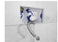
All moving parts can be removed through opening.
