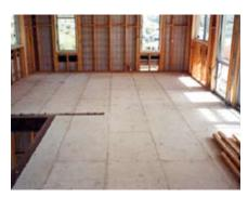
Figures 3.1, 3.2, 3.3 show typical applications for Hebel PowerFloor, for more details refer to Hebel Technical Update TU-009.
