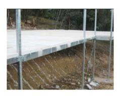
The floor applications consist of a Hebel PowerFloor panel connected to a steel or timber joist system forming a platform floor.
