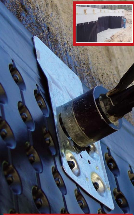
PLATON: A UNIQUE DOUBLE DIMPLED HDPE MEMBRANE INTENDED TO PROVIDE AN IMPERVIOUS BARRIER FROM LIQUID WATER FOR USE IN MANY APPLICATIONS
