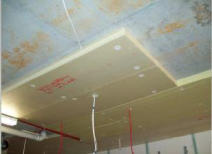
Foamular is lightweight yet tough and durable, it is easy to handle and quick to fit, saving on labor costs plus the need for extensive structural support and scaffolding.
