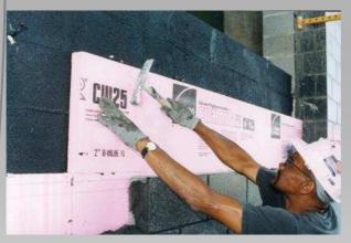
Foamular Extruded Polystyrene is closed celled insulation, so it is not effected by moisture. It can reduce the transfer of moisture and is its physical properties are not reduced in the presence of moisture.
