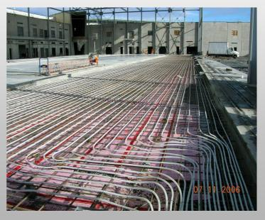
Fixing Foamular as a thermal barrier minimises heat loss so less energy is required to maintain slab temperature.
