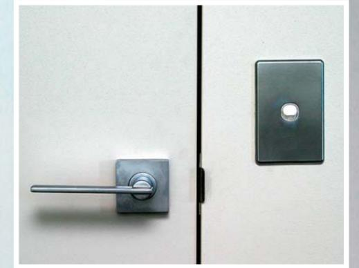
The completed jamb is flush finished and can be painted in with the whole wall area to fully conceal any fixing, achieving simple clean lines around the door face. The incorporation of reinforced edges overcomes the continual damage door jambs are subjected to by normal everyday use.
