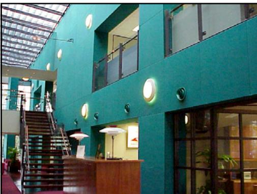
The on-site installation of the KlipTex® overcomes problems of prefabricated panels. Perfect alignment with adjacent architectural features and fittings is assured by the customised installation by factory trained personnel.
