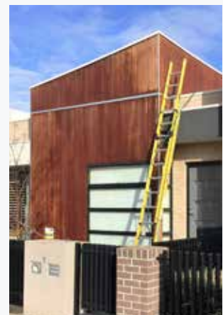
CLEANING: Wash the boards with a product like Intergrain Reviver or Cabots Deck Clean and a firm brush.
