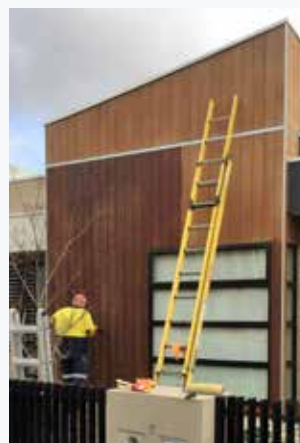
STAINING: Stain in the same direction that the boards run - vertical for vertical cladding.
