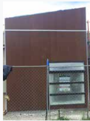
0 MONTHS: Recently built, this shows the beginning colour of Weathertex Natural boards.
