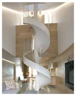
15.04mm low iron toughened structural laminated curved glass balustrade Engineered for compliance without a top rail
