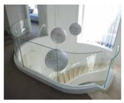
15.04mm Starphine toughened structural laminated curved glass balustrade. Engineered for compliance without a top rail
