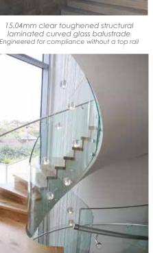
Inner balustade15.04mm clear toughened structural laminated curved glass
