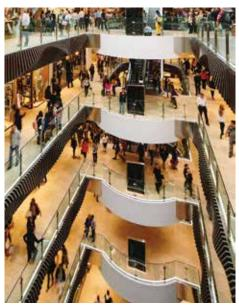
21.52mm clear toughened structural laminated frameless curved glass balustrade
