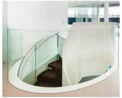
15.04mm clear toughened structural laminated curved glass balustrade Engineered for compliance without a top rail
