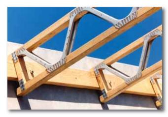
PosiStrut's innovative design also makes them ideal for roof construction. They can even be manufactured to create curved structures. Although popular in domestic construction, PosiStruts are now making a name for themselves in a vast array of commercial and light industrial applications because they offer a far more cost-effective solution to steel and are much easier to install. In fact, PosiStruts make excellent purlins, rafters...or floor joists!
