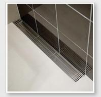
Wall to Tile The wall to tile drain runs along a wall and between a wall and tile or shower screen.
