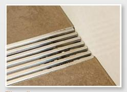
Tile to tile The tile to tile drain runs between two walls and has tiles on either side of the grate.
