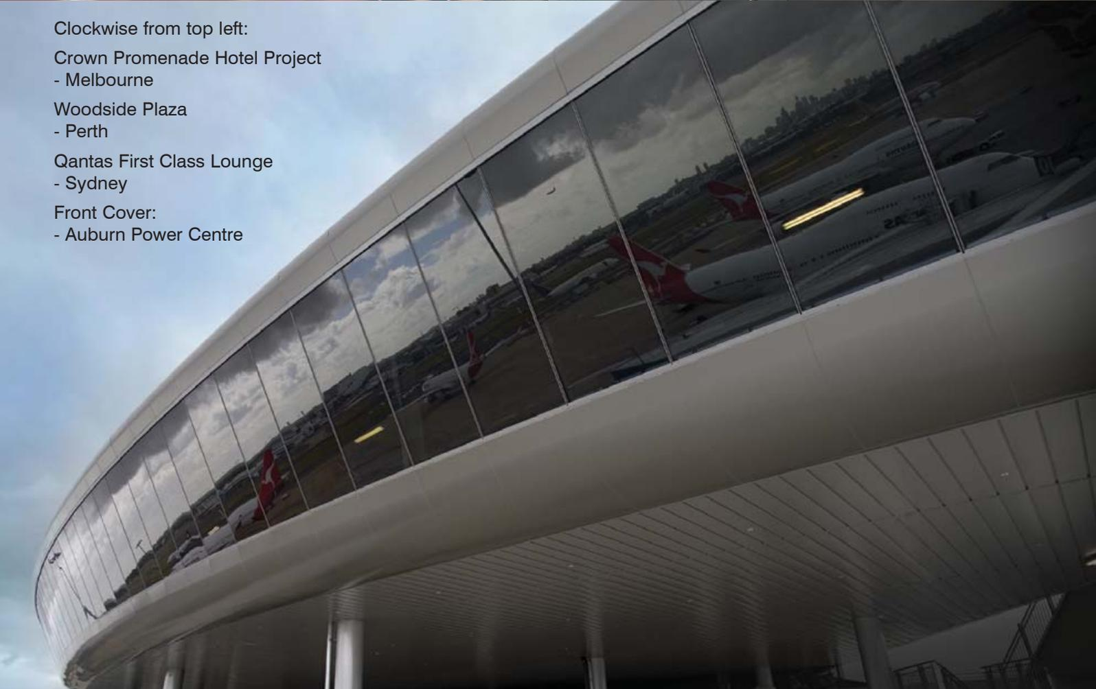
ALUCOBOND® is a light composite material consisting of two aluminium cover sheets and a core made of polyethylene. This simple but extremely versatile product concept has been developed to provide a façade material with a host of distinct advantages for architects: it is stable and yet flexible, has a smooth surface and is available in a number of standard or individual colours; it is weather-resistant, unbreakable, shock-resistant, vibration absorbent and easy to install.
