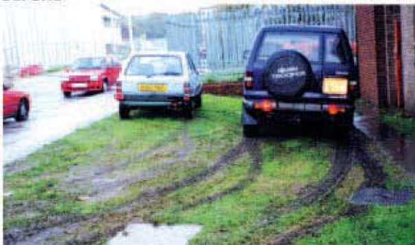
Roadside parking on unstable ground
