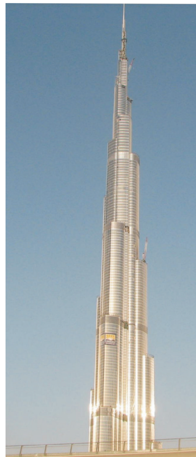
Burj Khalifa Tower used lagging technology acquire by Pyrotek that is used in Soundlag 4525C
