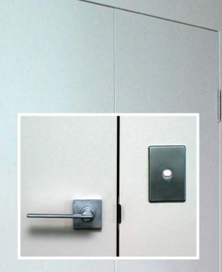
The completed jamb is flush finished and can be painted in with the whole wall area to fully conceal any fixing, achieving simple clean lines around the door face. The incorporation of reinforced edges overcomes the continual damage door jambs are subjected to by normal everyday use.
