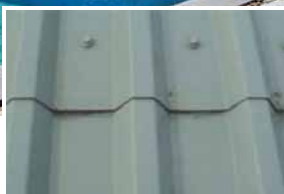
Colorcoat HPS200™ with Galvalloy™ roof after 7 years.
