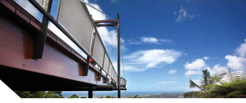
The platform projects a total of 21.6 metres from the promenade edge. Large section laminated beams (485x85) made from SE Queensland hardwood are supported by an innovative stainless steel cable structure. The decking is turpentine, the handrails grey gum.
