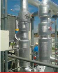
Closed cell, physically crosslinked polyolefin foam insulation with ultra tough foil facing to prevent mechanical damage in high risk areas.
