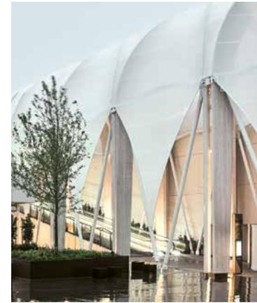
Starting from the arched glass roof of the Shopping Centre, we have designed a 110-metre long, arched passageway, which is based on a diagrid structure made from Italian larch glulam and topped with a stretch-resistant, semi-transparent PTFE canopy. Despite the openings in the edges of the structure, provided for cross ventilation, the design is extremely robust", describe the architects of "Make Architects" their Chadstone Link.
