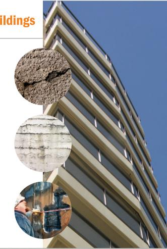
Other than poor aesthetic appeal, cracks in a buildings protective finish leaves the building vulnerable to premature masonry failures as the cracks allow the ingress of water, chloride irons, (salts), and environmental gases such as, (So2 and Co2) into the masonry substrate and expose the concrete and it's reinforcement to their potentially destructive effects.
