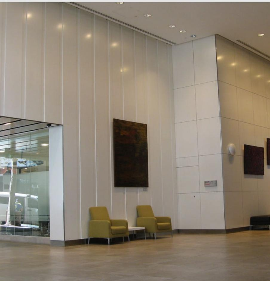
▼ SUPALINE grooved in 4 different spacings in durable SUPAFINISH Hoop Pine limed in a circulation area.
