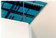
The unique design of SAS System 150 allows every full tile to pivot and slide along the grid system. The hinge and slide feature facilitates easy access to large areas of the ceiling void for maintenance; tiles are retained within the ceiling grid avoiding damage and eliminating the need for storage.
