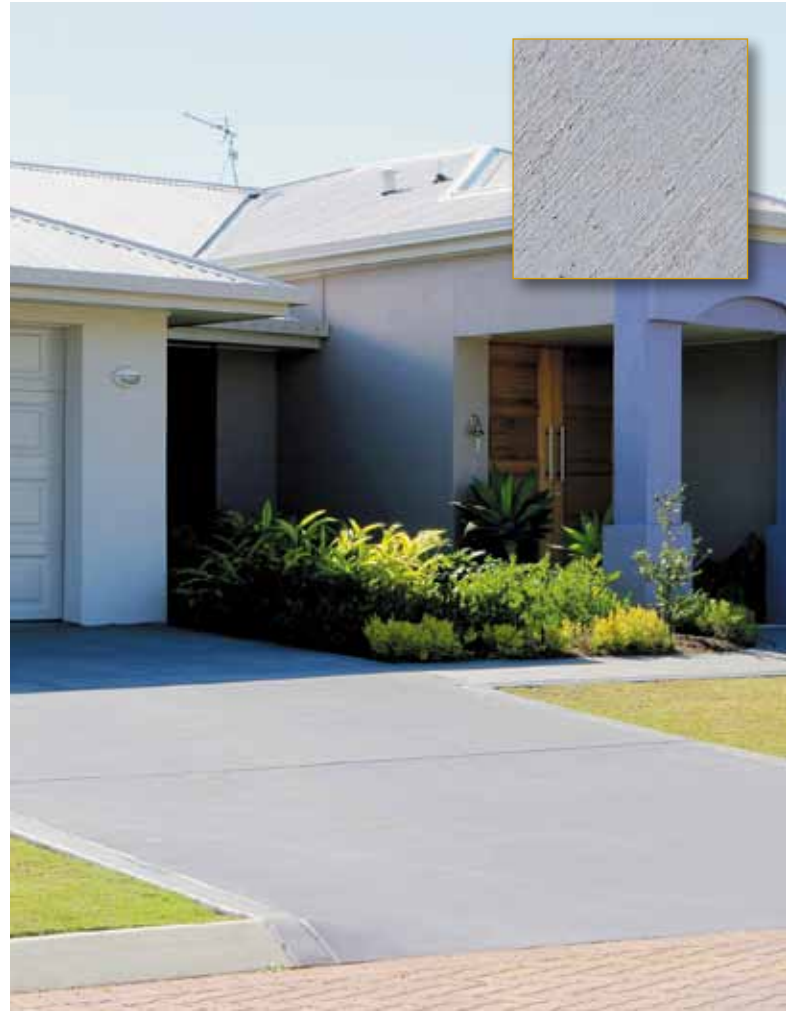
Below: Contrasting texture and colour is both a simple, yet highly effective way of creating an interesting driveway. Broom finish on the left with exposed aggregate to the right of the poodle. Colours: CCS Sandplain and CCS Onyx 21.
