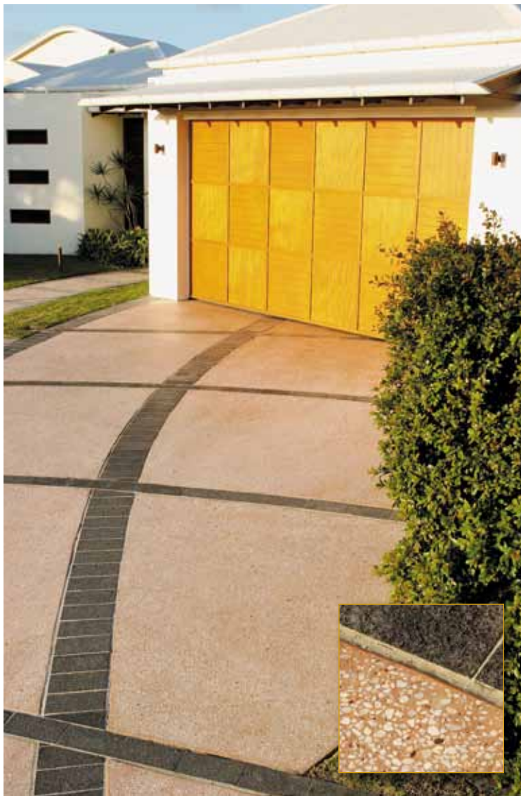
Above: Black pavers were used in the sweeping inserts. CCS Caramel was used to colour the concrete. The coloured concrete was honed to provide a smooth surface finish.
