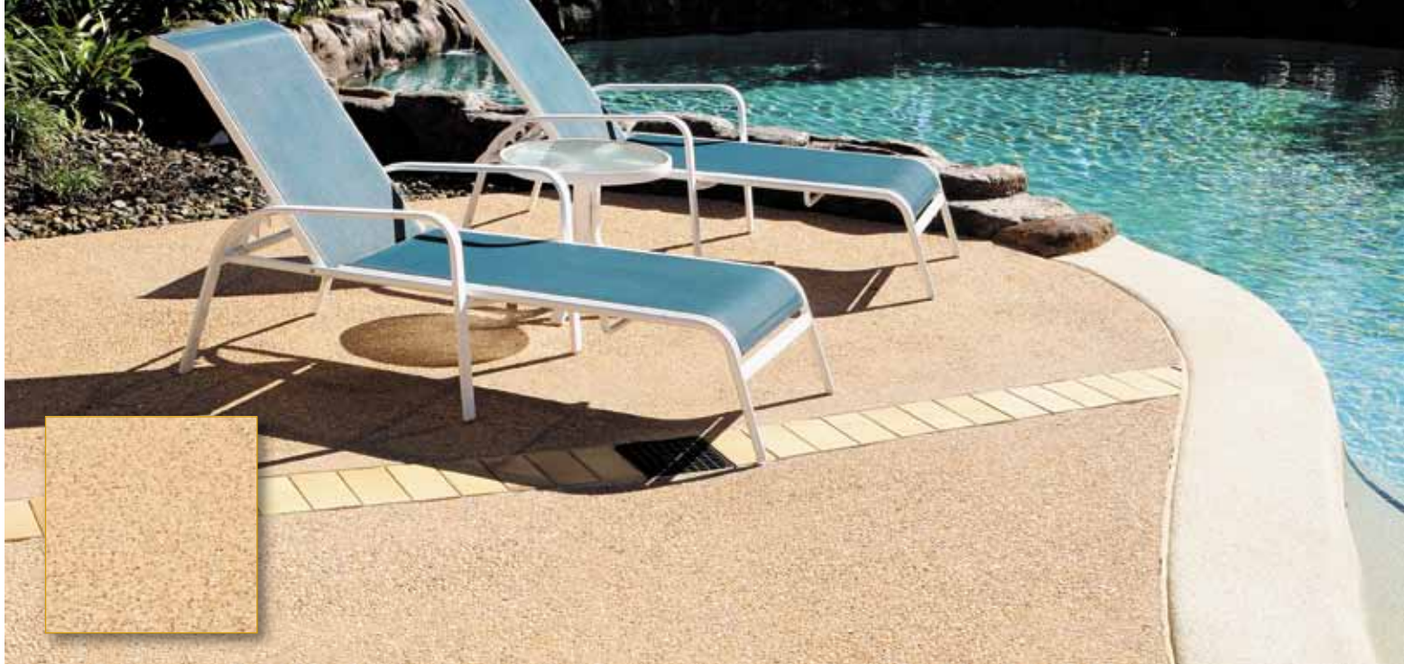
Above: A medium or lightly exposed coloured concrete finish is attractive, stable under wet feet and able to withstand the harsh environment of salt and chlorinated pools. Colour: CCS Biscuit, exposed aggregate finish.
