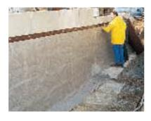
Layer 2: The polypropylene geotextile mat. Securely bonded to the dimple crowns by thermal welding, the mat provides excellent compressive stability and superb filtering performance. The rot-proof geotextile removes suspended soil particles and prevents clogging of the flow passages in the dimple texturing. The result: continuous drainage of incoming water to the take-off system below. Drainage capacity is further increased by the close dimple spacing of the new texturing pattern.
