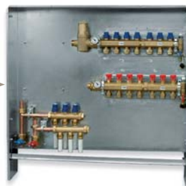
STAGE 2: installation of low- and high-temperature manifolds
