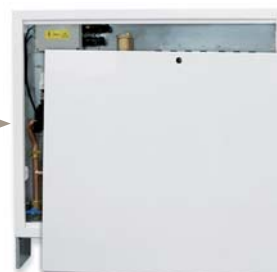
STAGE 4: installation of painted door and frame
