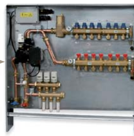
STAGE 3: installation of COMPACT mixing module/pump
