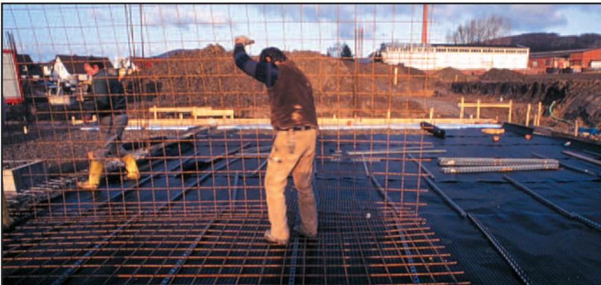
Reinforcing mesh and concrete are placed over the Platon membrane using standard placement procedures.
