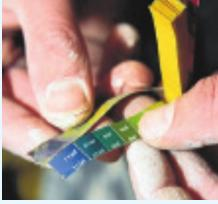
8. Litmus paper can be used to check the surface has been properly neutralized from the chemicals and will indicate when it's OK to paint.
