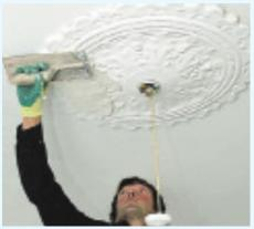
3. For larger areas a plasterers trowel can be used. Once paste is applied to the ceiling rose, go over it lightly with a brush to ensure there are no air pockets.
