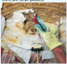
**6.** Use the spatula tool to pick away any stubborn parts of the paste, then you can give the surface of the rose a wipe down with steel wool to clean as much as possible.
