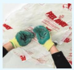
4. Cover the paste with the special Peel Away paper provided, masking sure there are no air pockets and printed side of paper is facing out.
