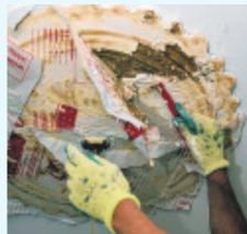
5. Leave the paste to work for up to 24 hours. Use the corner of the spatula tool to Peel Away the paper, which the paste and paint will normally stick to.
