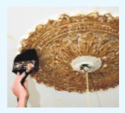
7. Once the paste has been removed, the surface is neutralized for future painting or residual chemical which could affect the new paint.
