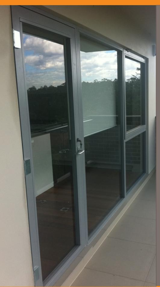
The Stopline E30 Glazed Fire Door is fully approved for fire ratings -/30/-. Designed and manufactured in Australia.
