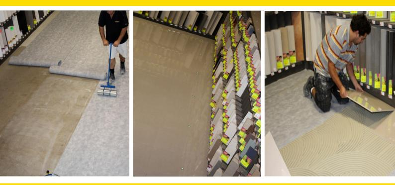
ARDEX DS60 Decoupling Mat is an inert Butynol<sup>®</sup> membrane based decoupling system for 'floating' floor tile applications. The system provides a hard wearing floor surface which can isolate any effects of the subfloor and at the end of its use can be easily removed without damaging the floor.
