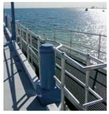
Weldlok<sup>®</sup> aluminium handrails and FRP walkway at Palm Beach Jetty, Rockingam, WA
