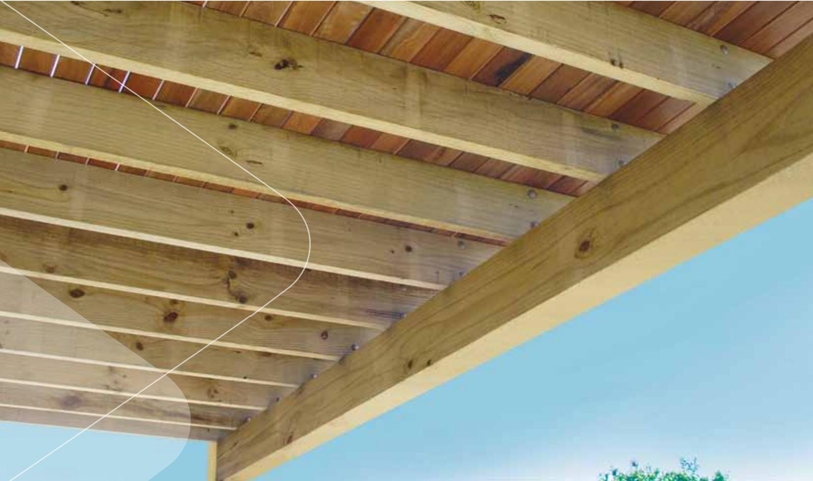
The selected MGP10 grade and unique H3 treatment makes Hyne T3 Green the new generation structural timber for external, above ground use. Offering a combination of guaranteed strength, improved stability, consistent reliability and outdoor durability, Hyne T3 Green provides real value for builders, architects, designers and for timber merchants who stock and supply outdoor timber.
