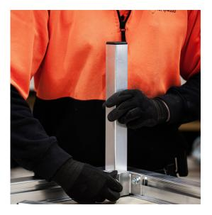
Insert the four Stage Legs and Hand tighten using the Wing Bolt.
