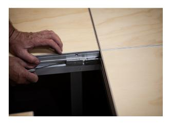
Insert Klemm-fix Connector the correct way up, going in just half way on Interior Podiums or the full way on Exterior Podiums.
