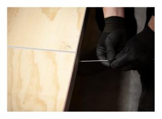
Lock the Klemm-fix Connector with the Allen Key Tool, Hand Tighten.
