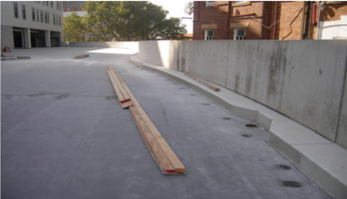
*Concrete curbing placed on 5mm Projex Shockmat membrane protection layer*
