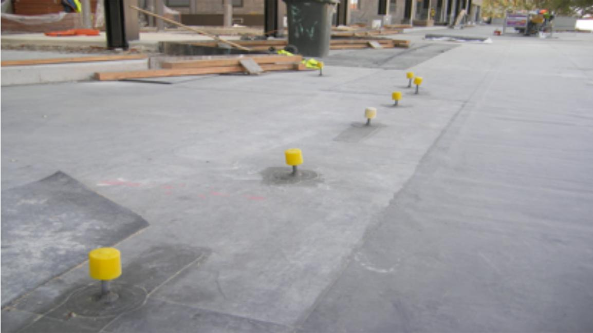
*Anchor points for concrete curbing and islands have been detailed & waterproofed using standard Wolfin installation procedures. Over 3,500 square metres of Wolfin were used in this area.*
