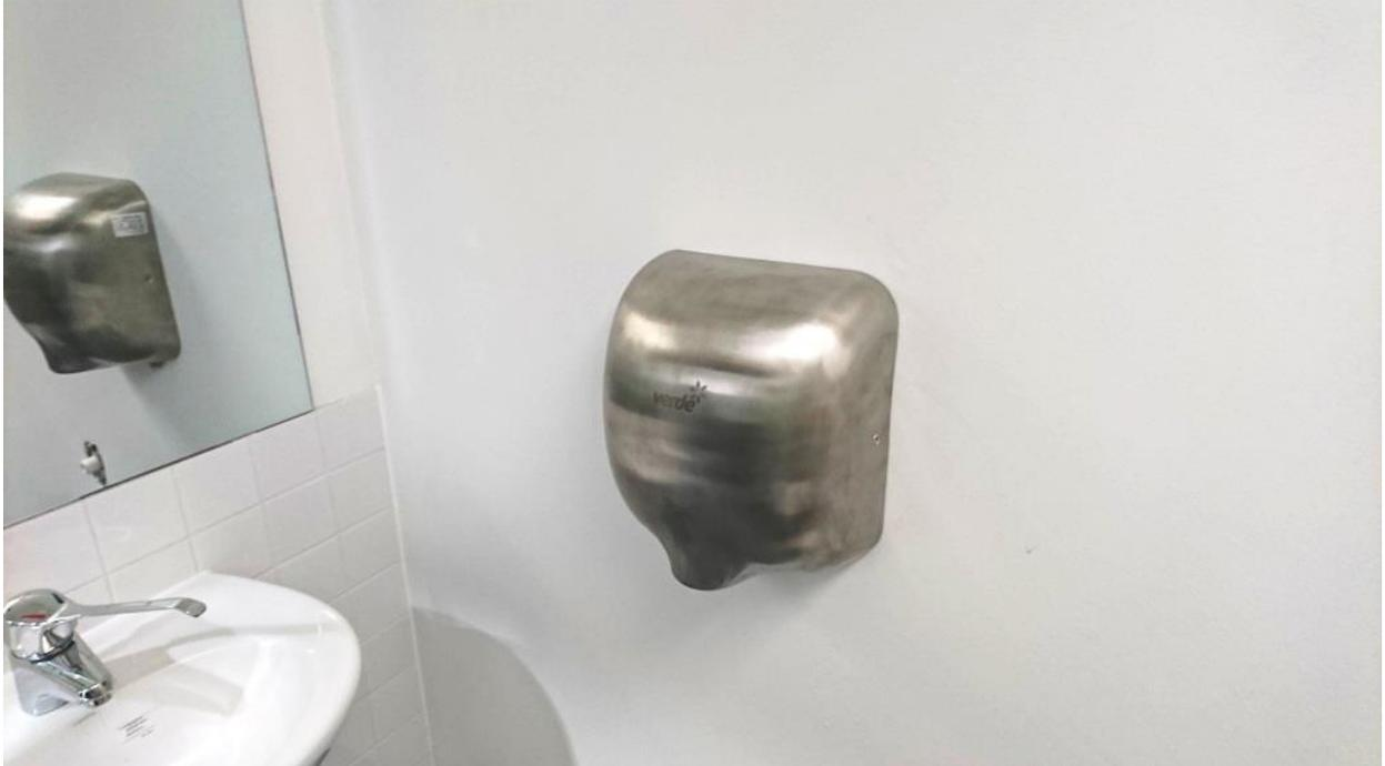
2. The operation sensor is situated on the underside of the unit, along with the air discharge outlet which is designed to concentrate the high volume, warm air onto the user's hands, quickly & efficiently drying excess water. The tamper proof, robust design lends itself to low maintenance requirements, with low running costs.
