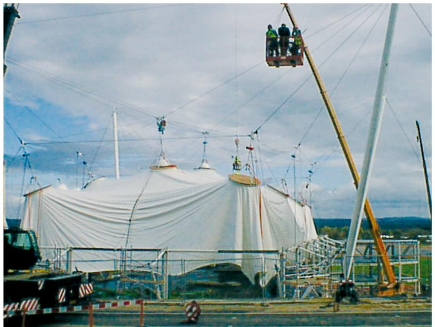
Installation phase for a high point shaped membrane roof. This process requires to be integrated into planning phase and must be carefully synchronized in the whole installation
