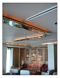
KlipTex<sup>®</sup> is a customised stretch fabric system which includes a sound absorption material concealed within the perimeter of the KlipTex<sup>®</sup> frame, over which the decorative fabric is stretched and locked in position.
