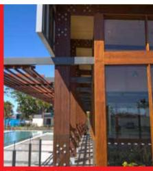
Hynebeam 17 is the strongest softwood glue laminated beam available, and suited to a variety of structural applications, particularly in high load, long span applications where performance is critical.
