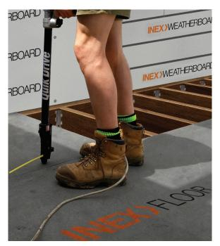
Figure 5a Alternative method of screwing INEX>FLOOR to steel or timber joists using freestanding screwing system
