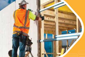
MaxiWall is a strong yet lightweight walling panel made from Autoclaved Aerated Concrete (AAC) and reinforced with corrosion protected steel mesh.
