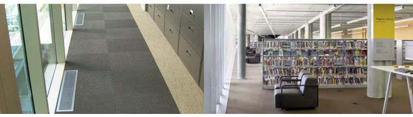
Segmented In-floor Active Chilled Beam application
