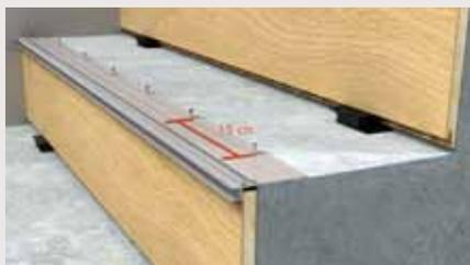
2. Glue and screw the aluminium sub-profile on the step.
