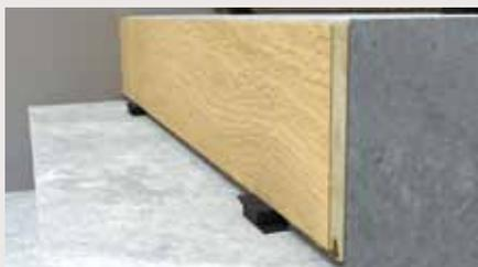
1. Glue the plank to the riser. The spacers ensure that sufficient space is left underneath to fit in the step.
