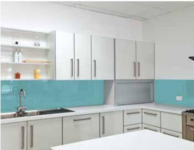
Zenolite panels can be fabricated and cut on-site by the installer, allowing custom fitting to out of square walls and accurate location of cut outs for power and water points.
