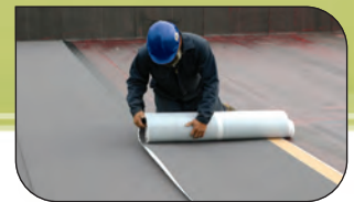
Finish with cap sheet membrane
