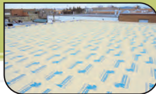
Vapour barrier installation
