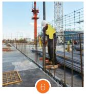
Core filled via a boom pump sees walls become load bearing
