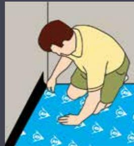
Roll out the selected Dunlop hard flooring underlay and trim any excess so that the ends and sides fit neatly against all walls.
