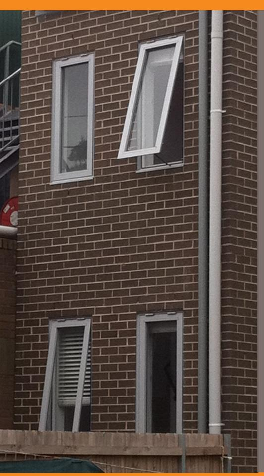
The Autofire auto closing fire rated window system is fully approved for fire ratings up -/60/-. Designed and manufactured in Australia.
