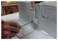
Ensure that the overflow is properly connected before the benchtop is installed. The overflow must be factory fitted – once the benchtop is installed on-site there is ordinarily nil access for fitting of overflow to rear of sink.
