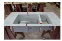
Clearance to front edge of benchtop: remember to account for the sink wall thickness being 24mm due to the strap on front of sink.
